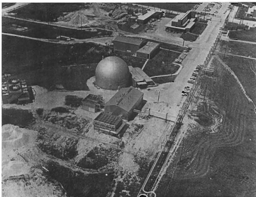
The Experimental Boiling Water Reactor Facility As Modified for 100mW Operation
